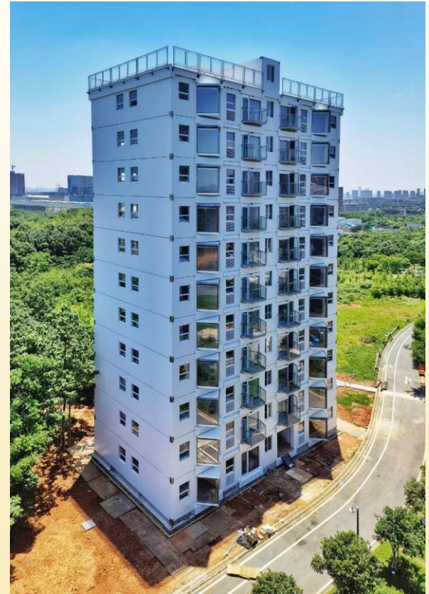
Completed in just 3 days
