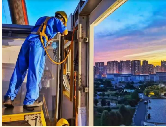
Bolting the exterior walls
