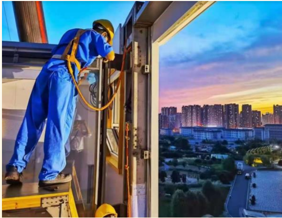
Bolting the exterior walls
