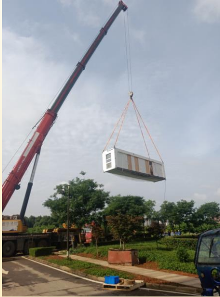
The beginning... the first module
