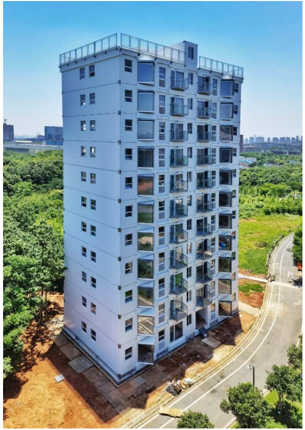
Turnkey Building stacked in 28 hours
