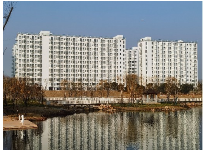
Fig. 4. BROAD Holon Building: Prefabricated stainless steel buildings produced to industrial scale
