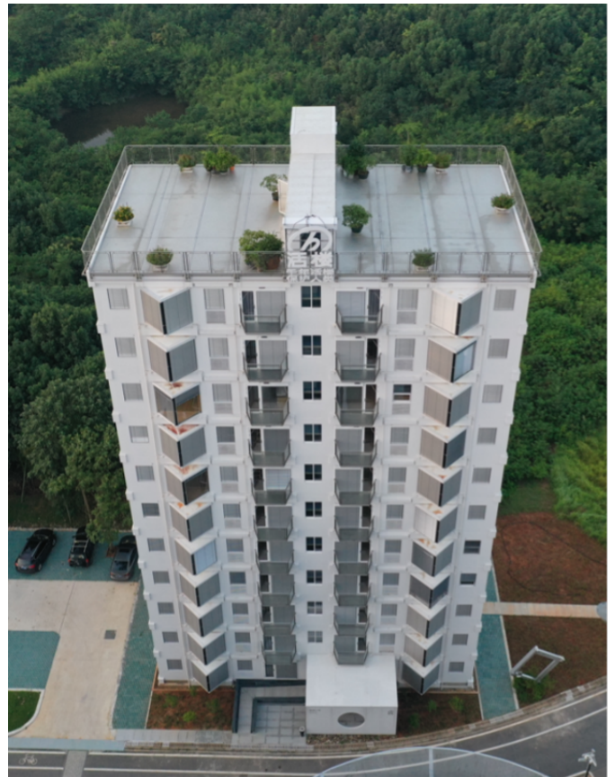
Fig. 5. BROAD Holon Home Garden Building: All load bearing structural members are composed of stainless steel
