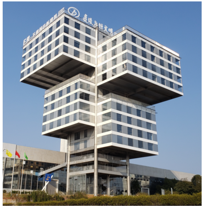
Fig. 1. BROAD F Tower: the first all stainless steel high-rise building
